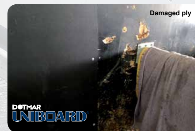
Dotmar Uniboard panel replacement of plywood at Warwick Farm Racecourse - NSW
